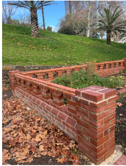
Figure: Low perimeter brickwork fence (rebuilt 2000)
