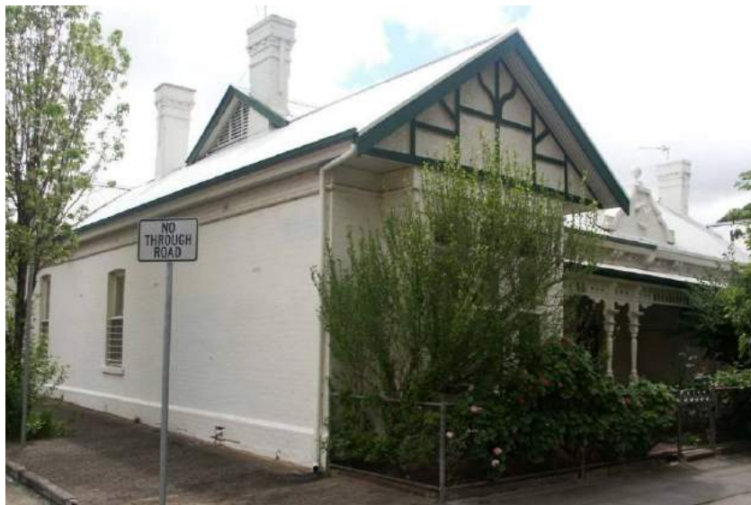
Villa, 394 Gilles Street — View to northeast
