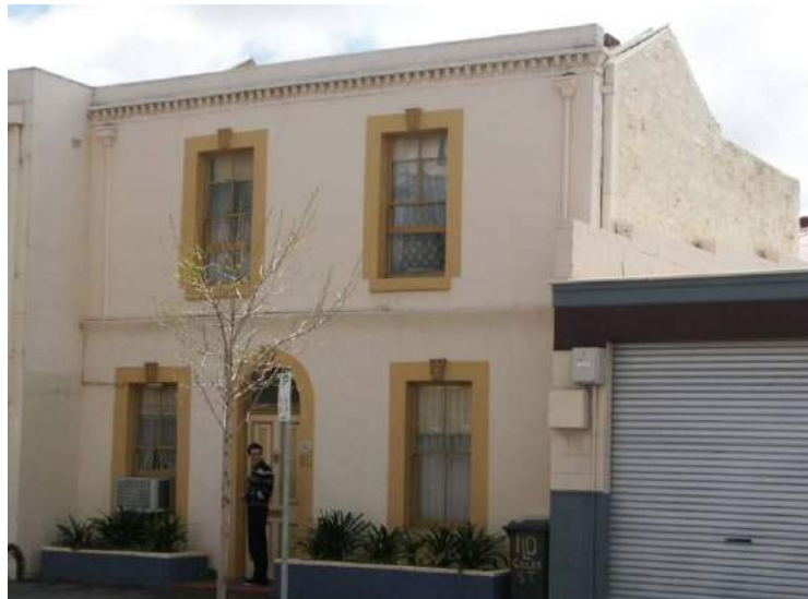
Albert House, 110 Gilles Street — View to northeast
