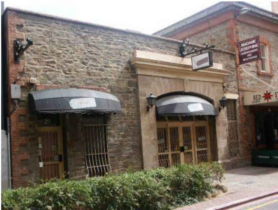
TMVC House, 27-39 Gilbert Place—View to northwest
