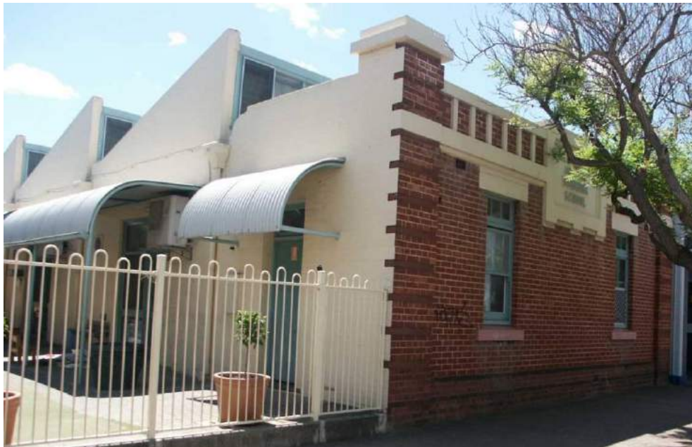
Child Care Centre, 102-106 Gilbert Street — View to northeast
