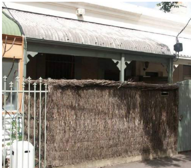
Attached cottage, 293 Gilles Street — View to southwest
