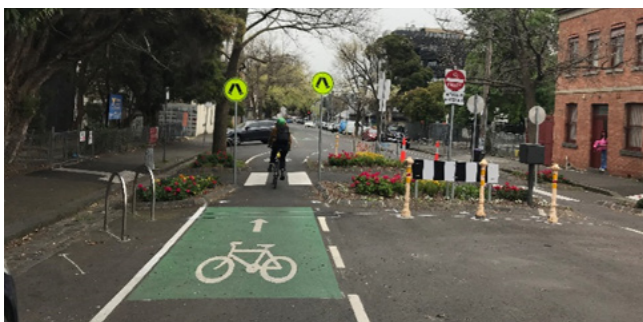
Modal filter adjacent to Fitzroy Primary School, Melbourne.
