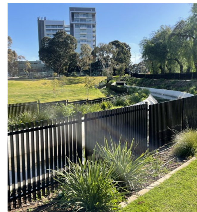
Concrete swale and fencing
