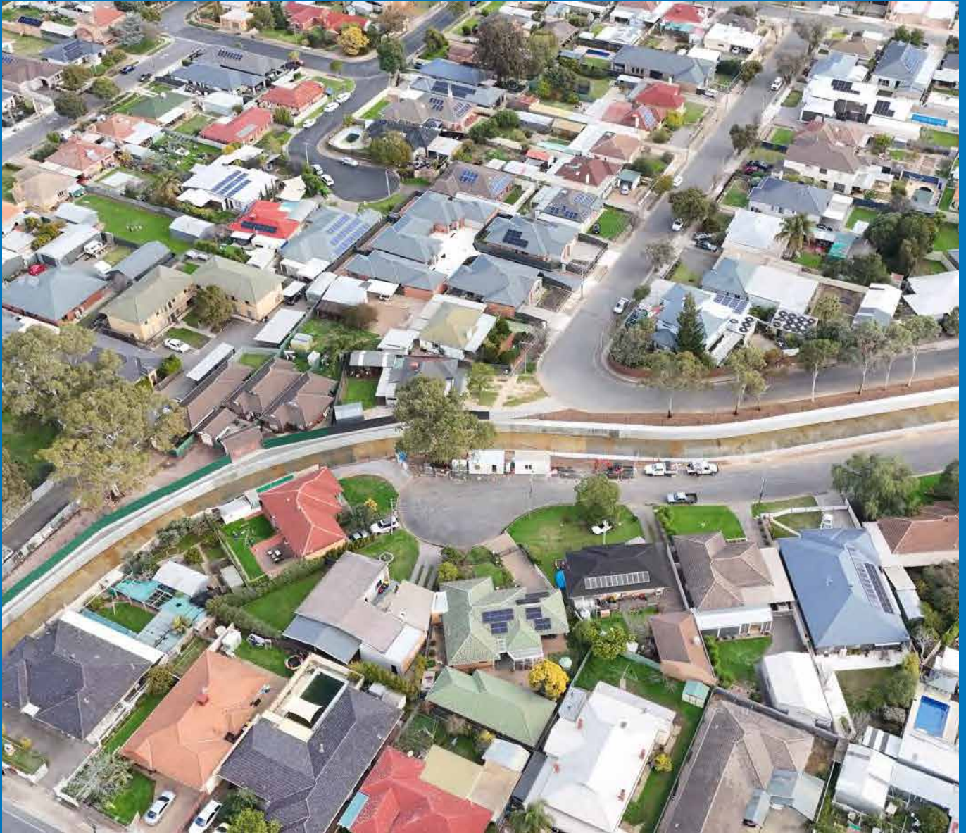
Lower Brown Hill Creek Upgrades
