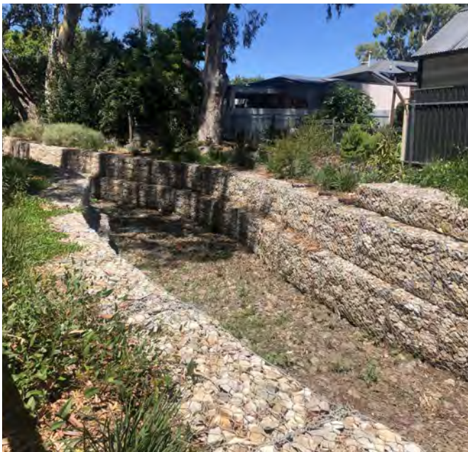
Rock filled gabions
