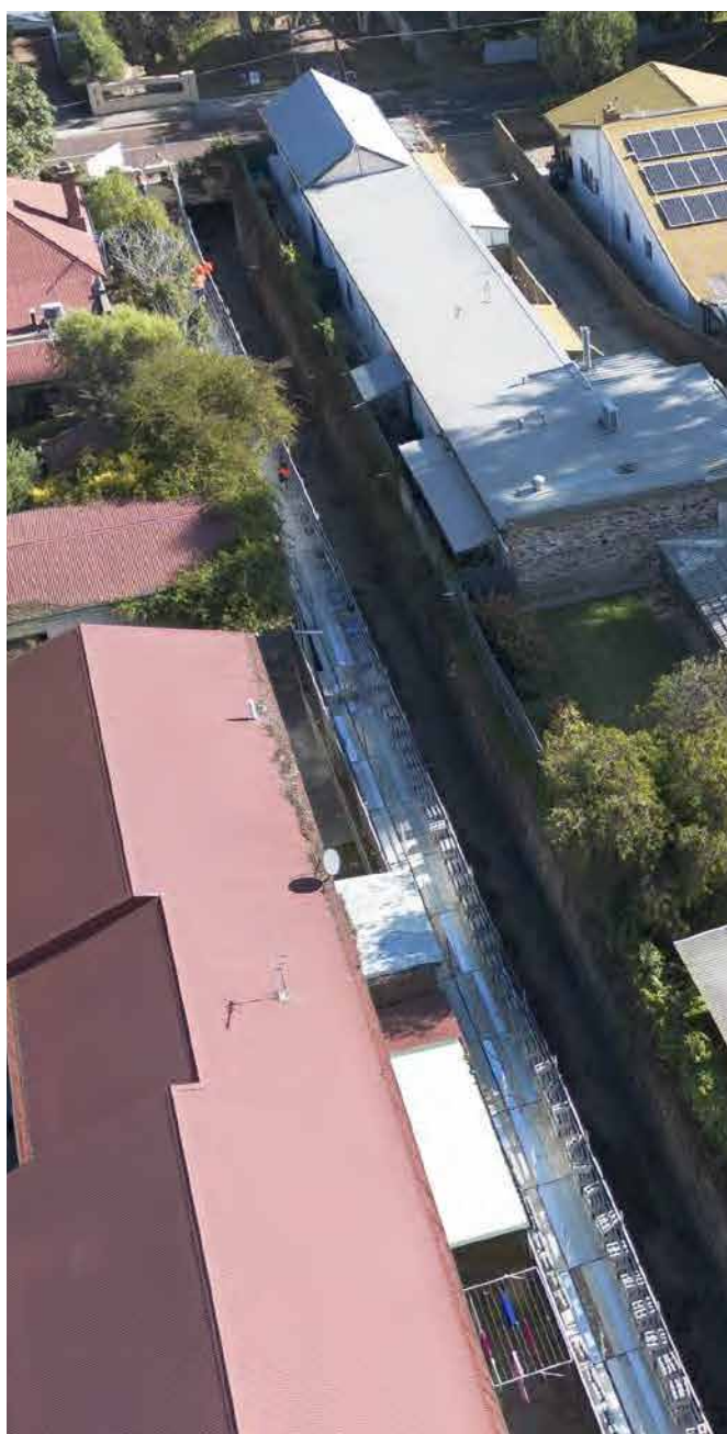
Leah Street to Ethel Street Channel Construction
