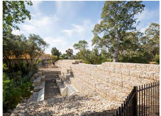
Flood Control Dam
