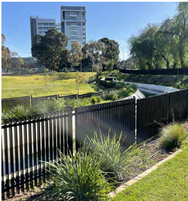
Concrete swale and fencing
