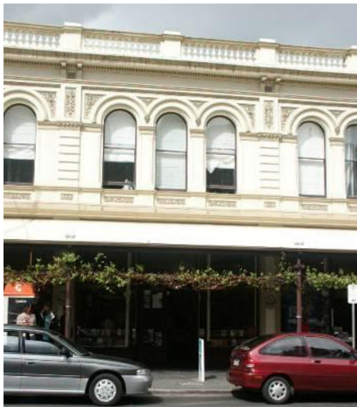
Shop, 107 Hindley Street – View to south
