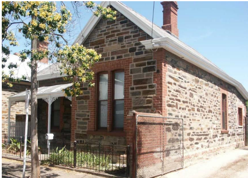
Villa, 11-13 Kate Court — View to northwest
