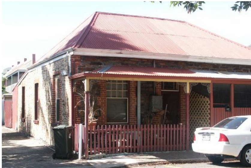
Attached cottage, 12 Weil Street — View to southeast
