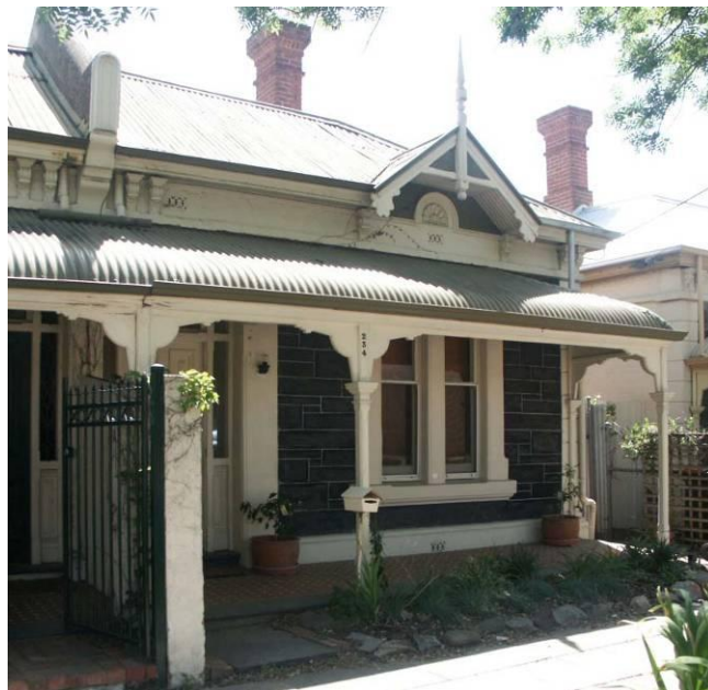
Attached villa, 232-234 Halifax Street — View to northeast
