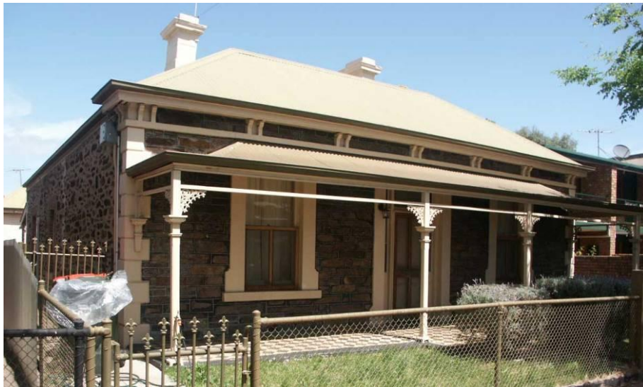
Villa, 265 Carrington Street — View to southwest
