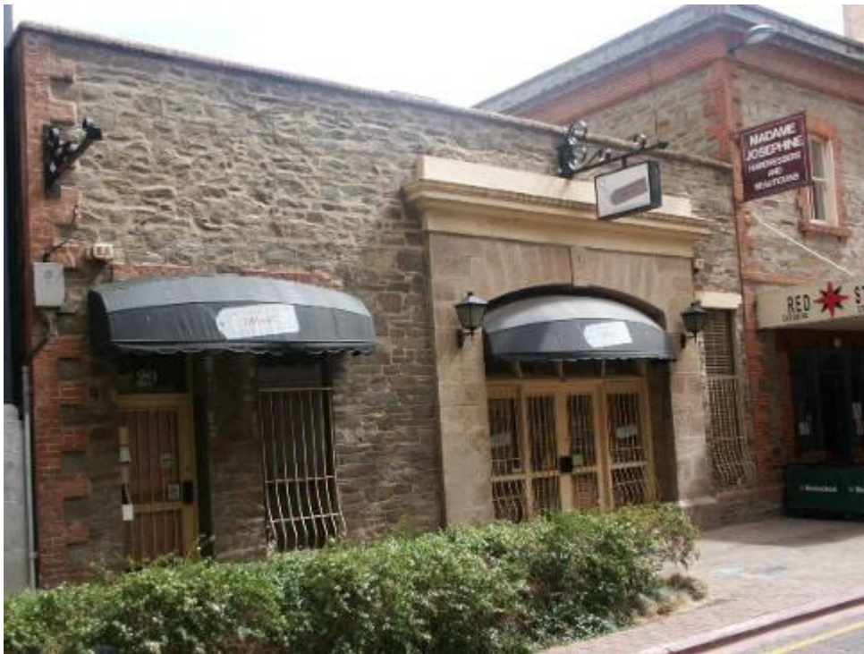
TMVC House, 27-39 Gilbert Place—View to northwest
