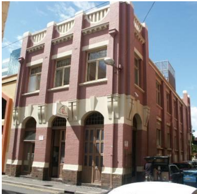
Commercial premises—View from Twin Street, to northeast
