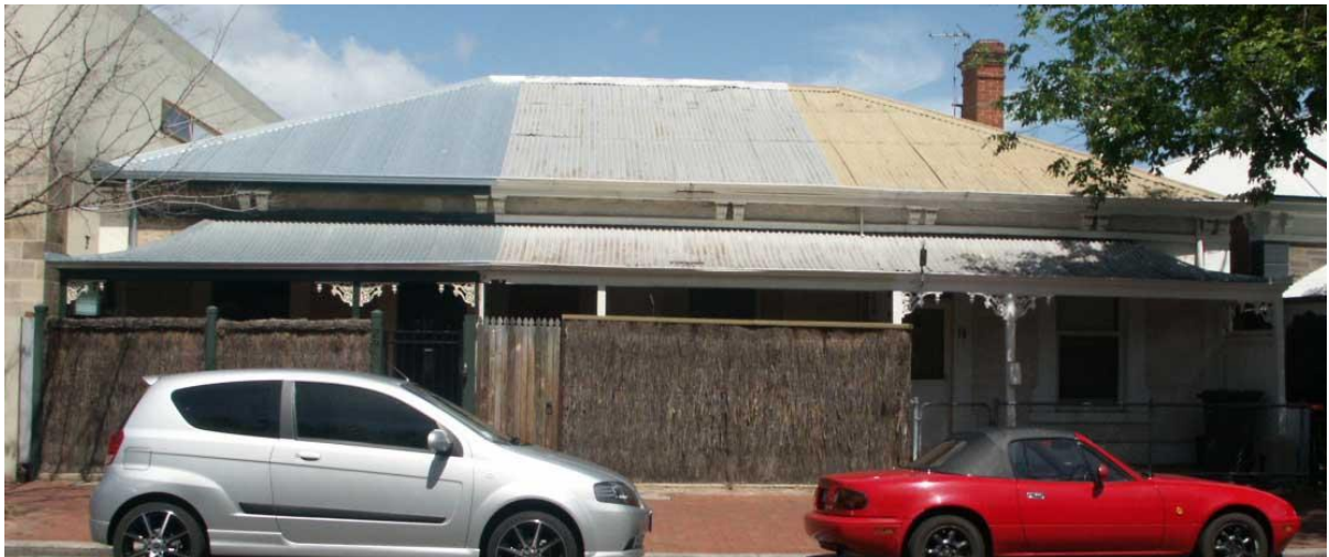
Attached cottage, 293 Carrington Street — View to south
