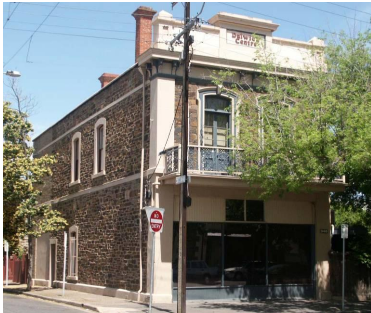
Dulwich Centre, 345–349 Carrington Street — View to southwest
