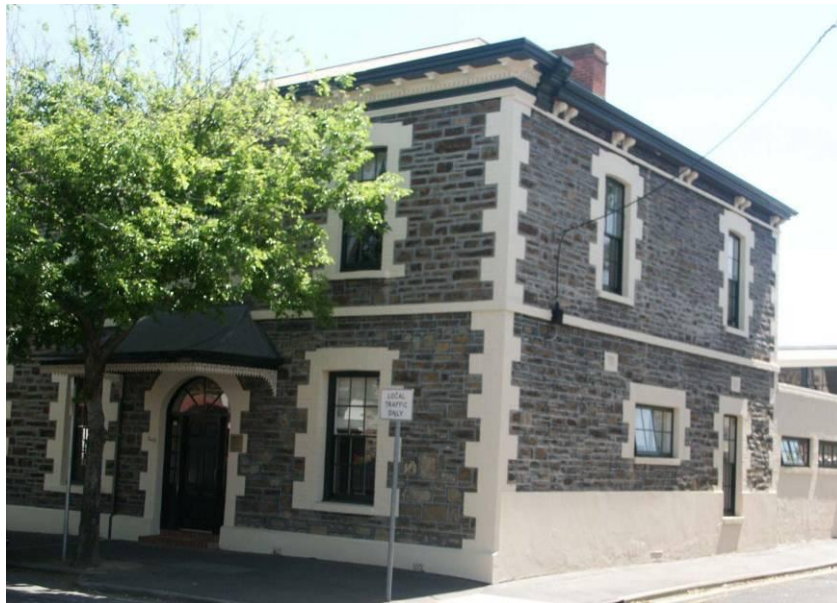
Offices, 346-350 Carrington Street— View to northwest
