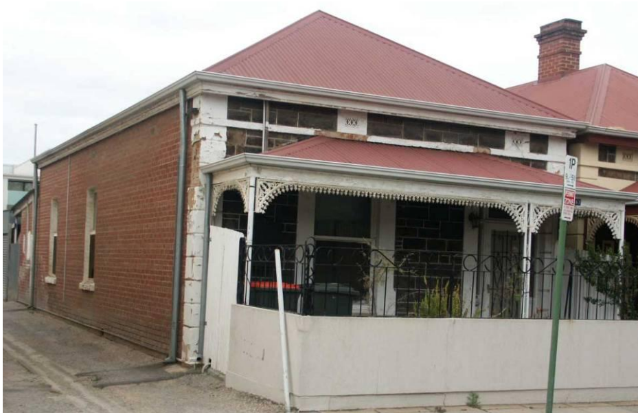
Cottage, 67 McLaren Street — View to southeast
