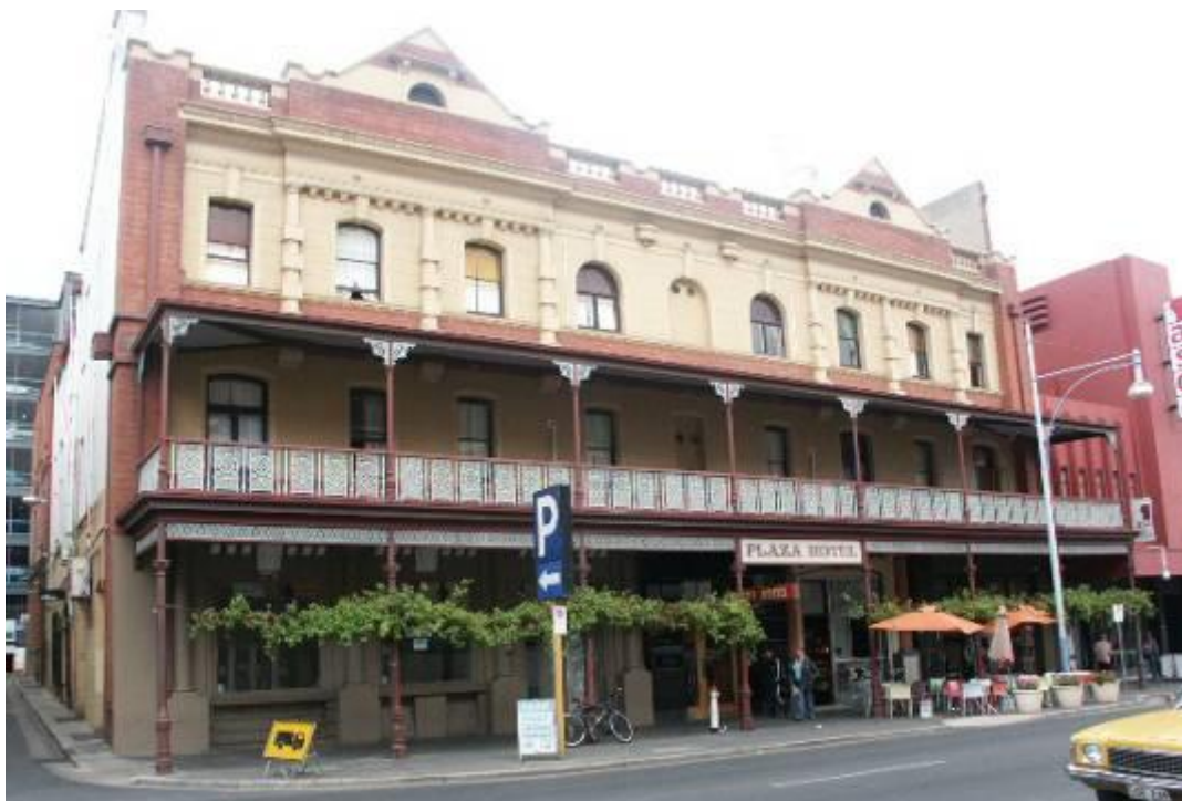
Plaza Hotel, 81-89 Hindley Street—View to south
