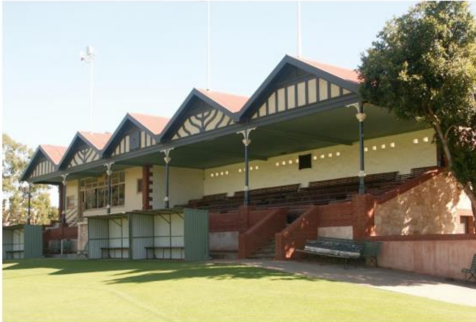
University of Adelaide Grandstand from oval (from east)
