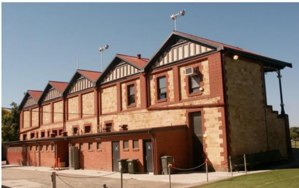
University of Adelaide Grandstand from rear (from west)
