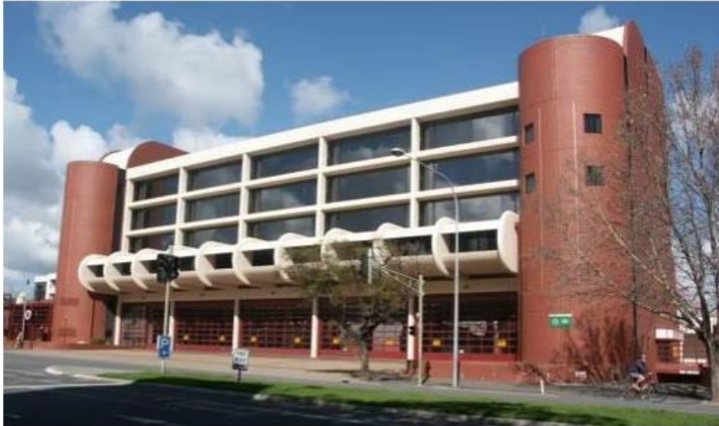
Adelaide Fire Station, 81-129 Wakefield Street Adelaide, View from north (Hamish Angas, July 2014)
