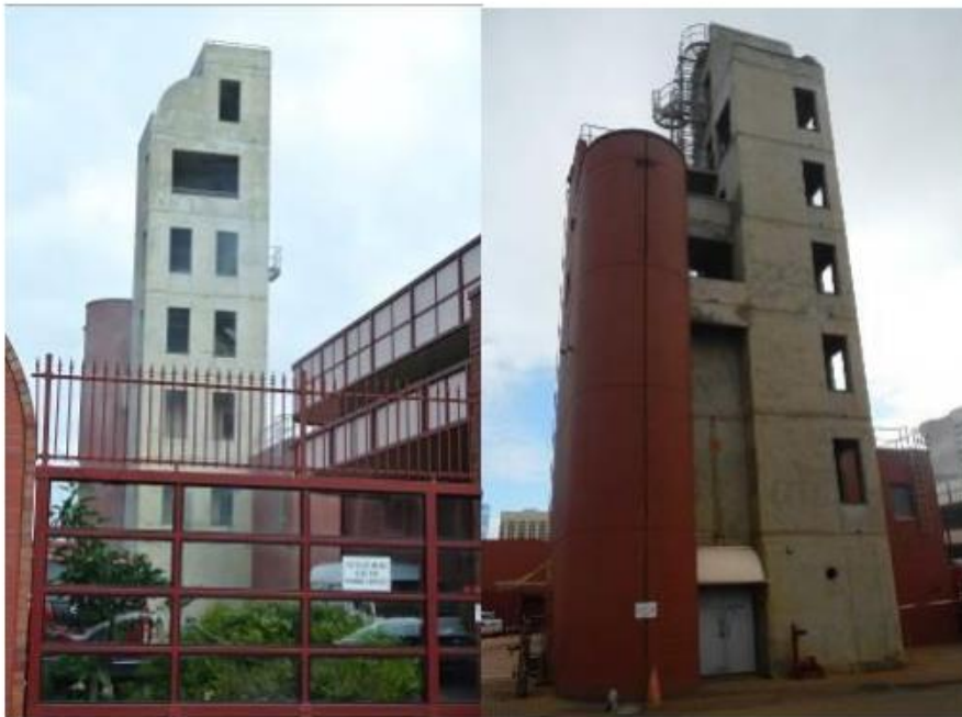
Adelaide Fire Station, 81-129 Wakefield Street, View of training tower from north & east (Hamish Angas, July 2014)
