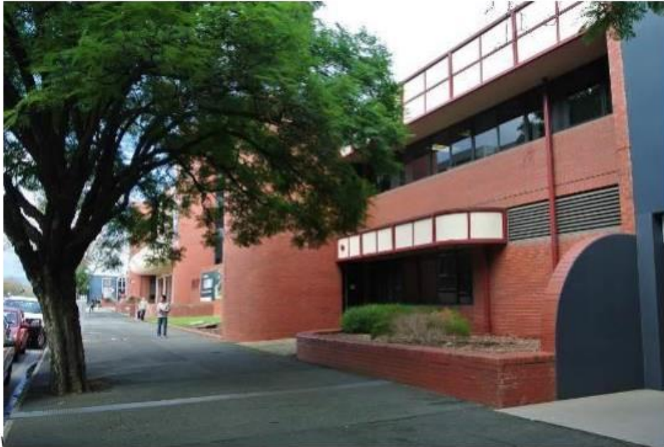
Adelaide Fire Station, 81-129 Wakefield Street Adelaide, View of western office building from north-west (Hamish Angas, July 2014)
