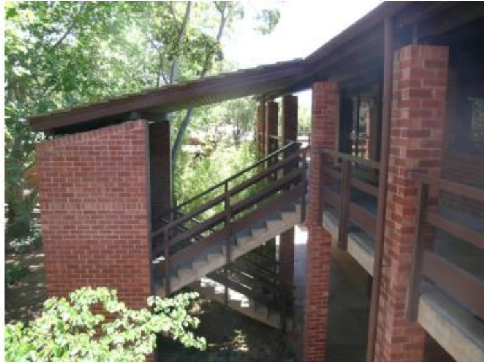
Amenities wing and stair, looking north (image: Hurst 2009)
