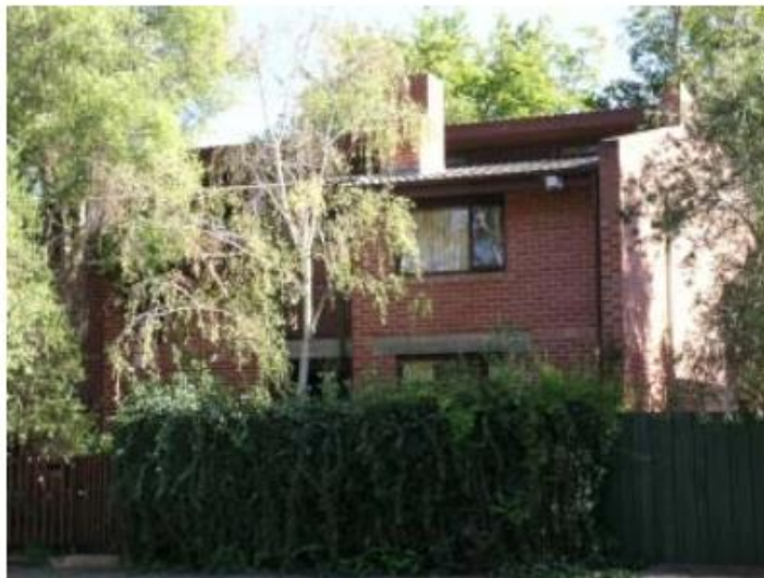
Master's House, Mackinnon Parade elevation, looking north (image: Hurst 2009)
