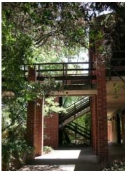
Entry from Mackinnon Parade: Amenities wing on right, looking north. (image: Hurst 2009)
