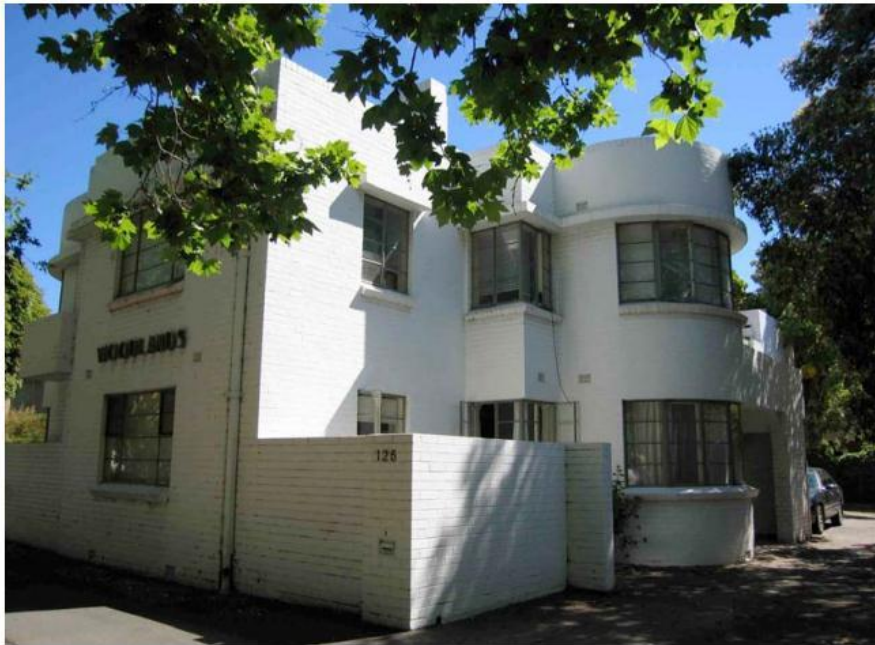
Woodlands Apartments looking south-west
